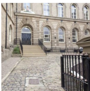
The Courthouse Bradford, UK
